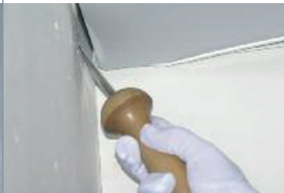
Fitting the ceiling with the CILING®-spatula
