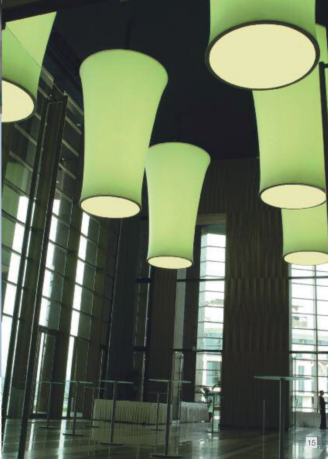
Palace of Arts Ludwig-Museum Budapest Highlight: 6 hanging lamps, Outer skin Luxell foil, upper \phi 2,50 m, lower \phi 1,65 m, funnel height 4 m, RGB-Control. The lower sides can be removed for maintenance.
