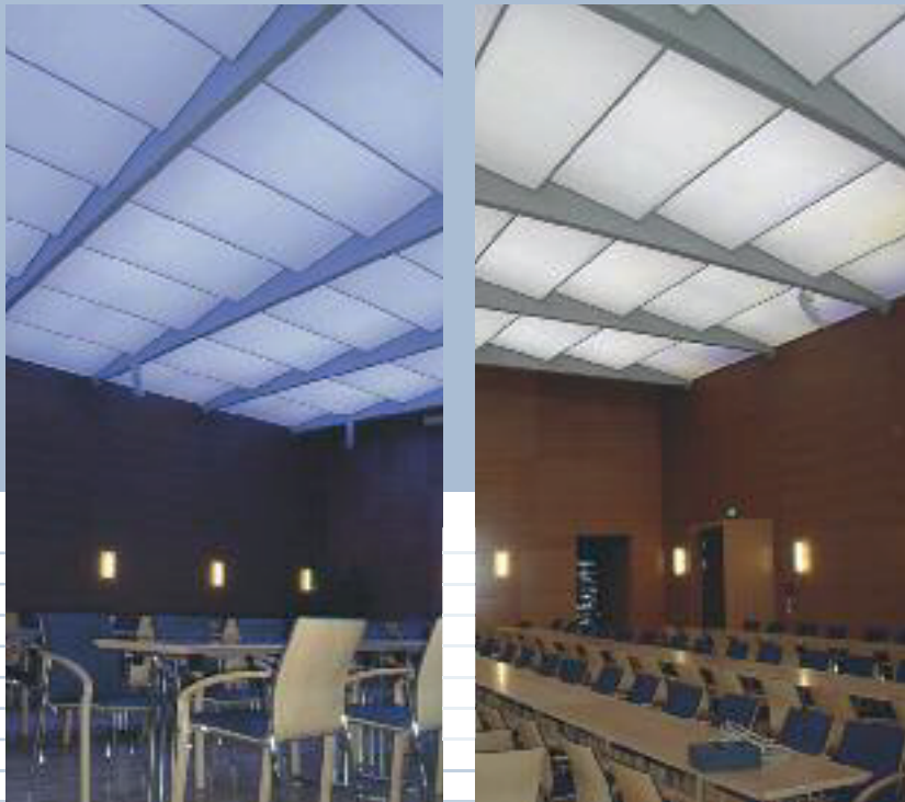
Miele showroom , headquarter Gütersloh – ca. 20 RGB-lighted ceilings create a light atmosphere in every color desired. Adjustable rim construction with a pull-out rope and RGB-T5 light control via a BUS system
