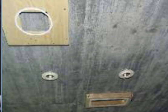
Sub-construction for the built-in lighting are fitted
