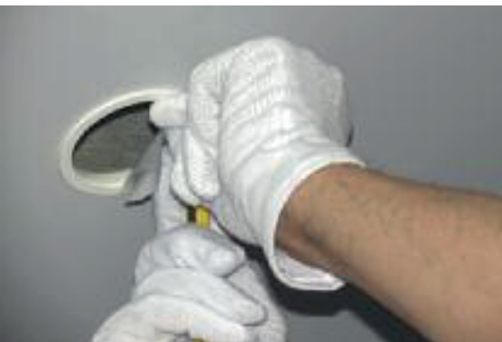
Cutting away the vinyl on the inside of the ring
