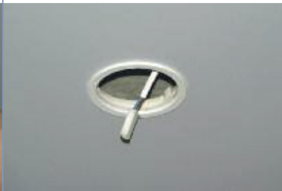
Opening for installation of lighting
