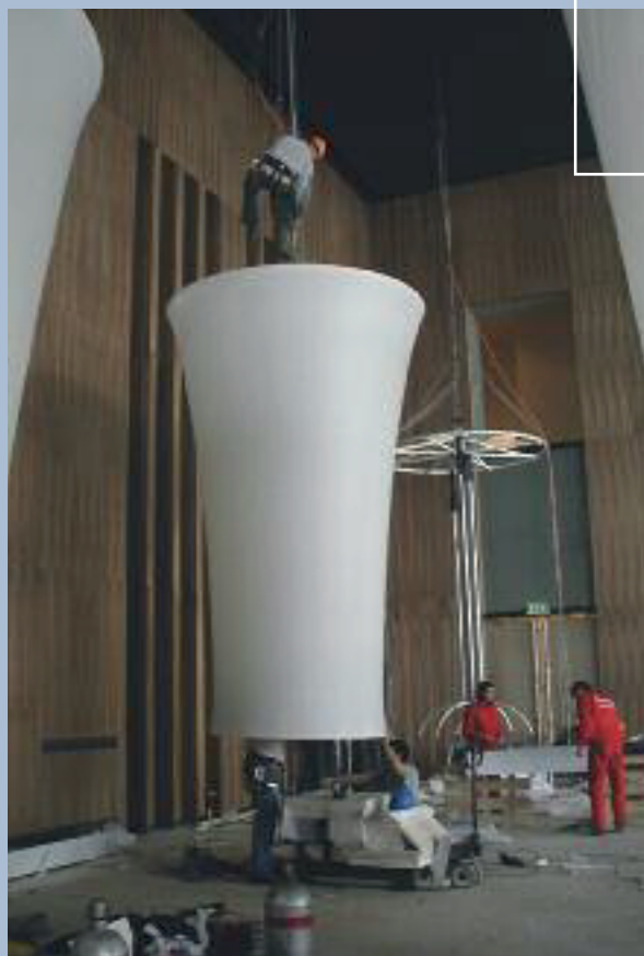
Palace of Arts Ludwig-Museum Budapest Highlight: 6 hanging lamps, Outer skin Luxell foil, upper \phi 2,50 m, lower \phi 1,65 m, funnel height 4 m, RGB-Control. The lower sides can be removed for maintenance.
