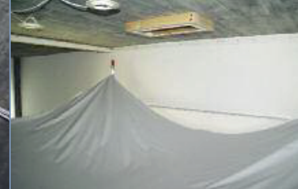
The stretched ceiling is clamped at all corners
